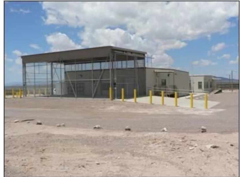
Deming, NM Forward Operating Base
