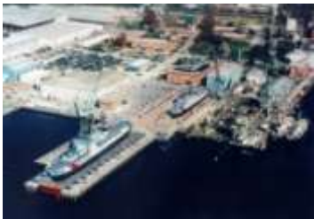
Industrial Facilities & Bases
