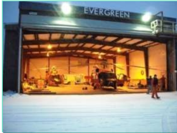
Cold Bay Hangar
