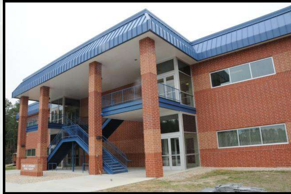
Dining Facility, Fort Lee, VA
