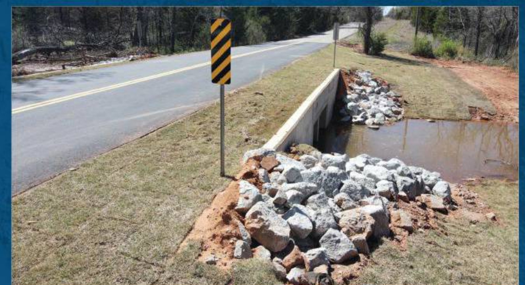
Post construction of one of the parallel headwalls showing the improvements to roadway safety and slope stability improvements.
