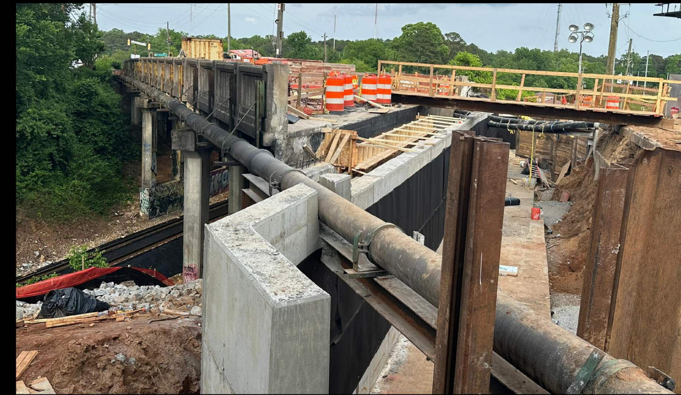
▲ A photo during construction showing temporary support for 12-inch watermain going through vertical abutment wall.
