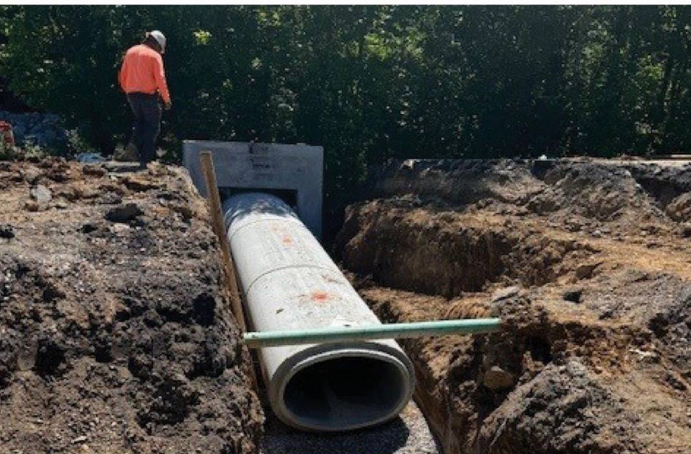
Drainage structures were field-modified to avoid utility conflicts.
