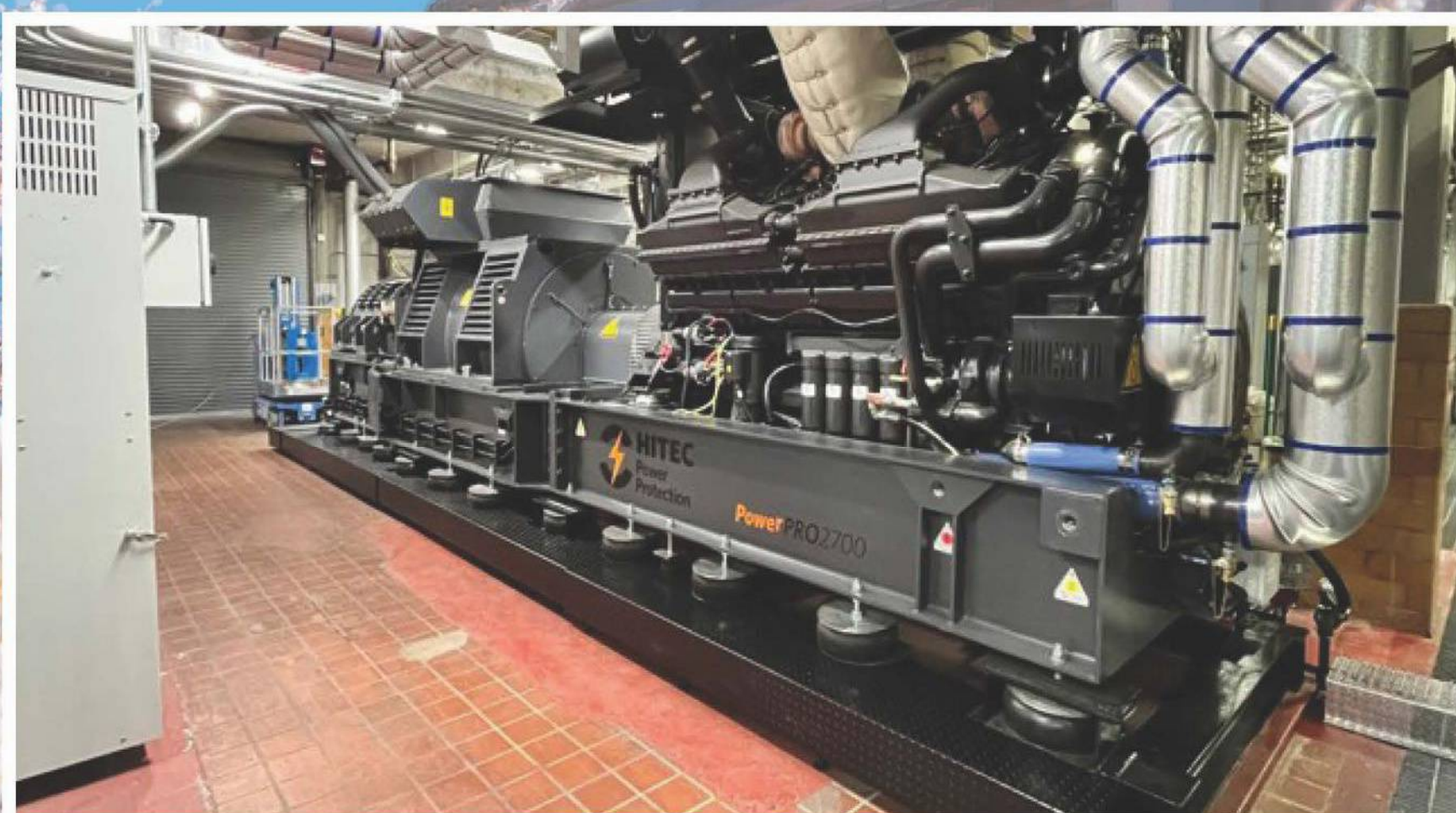
The DRUPS keeps the plant operational through short outages or, during longer outages, jumpstarts a diesel engine to keep the plant running.
