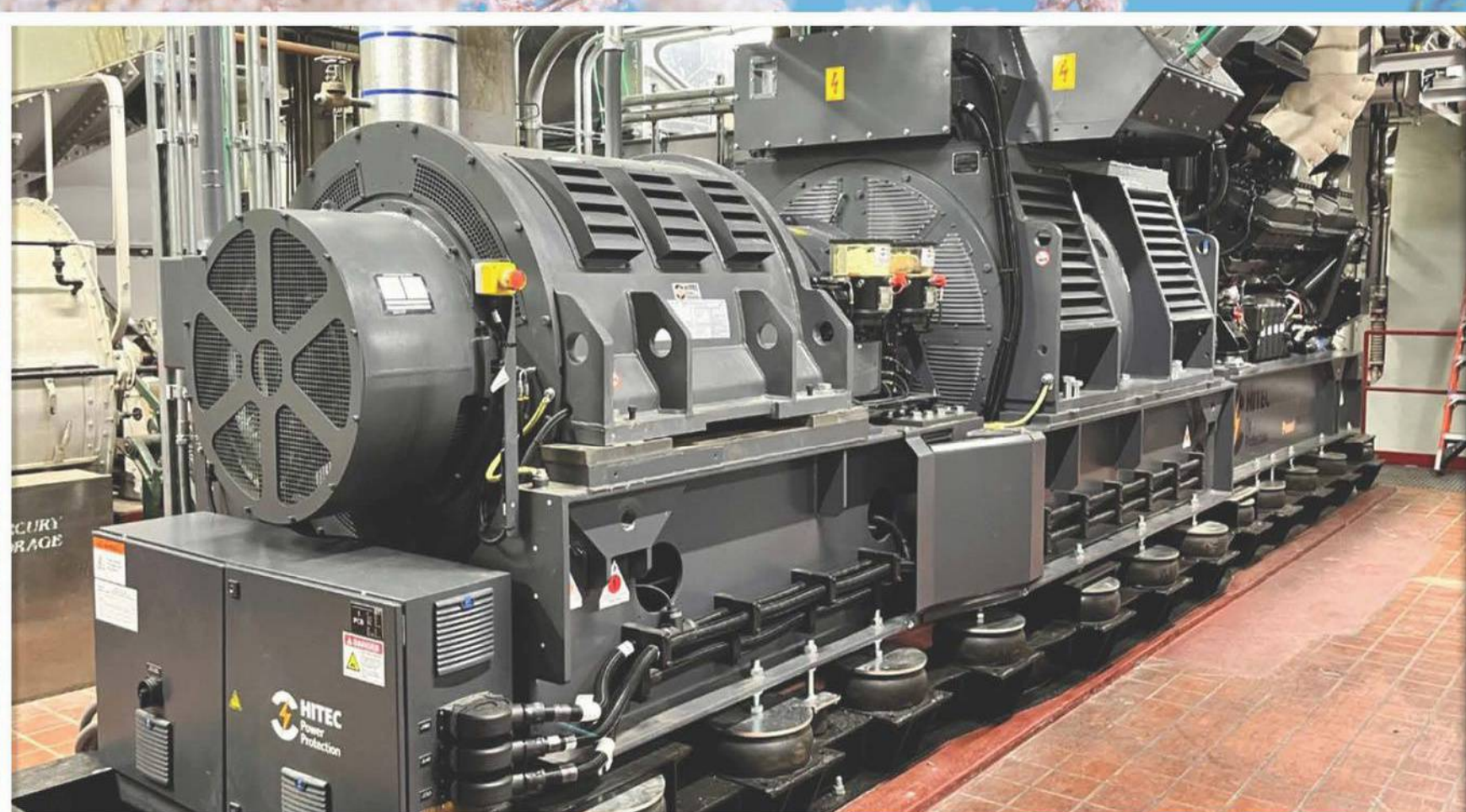
The University of Washington is thought to be the only US campus to employ a Diesel Rotary Uninterruptible Power Supply (DRUPS).
