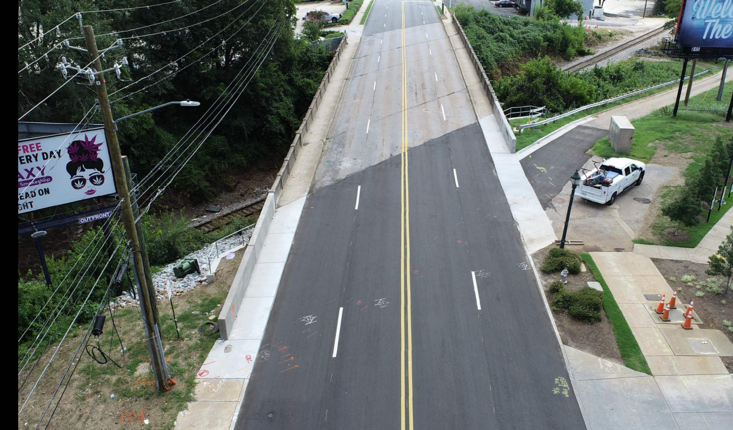
▲ An aerial image of the completed repair showing removal of damaged end span, construction of vertical abutment wall and its close proximity to CSX railroad.
