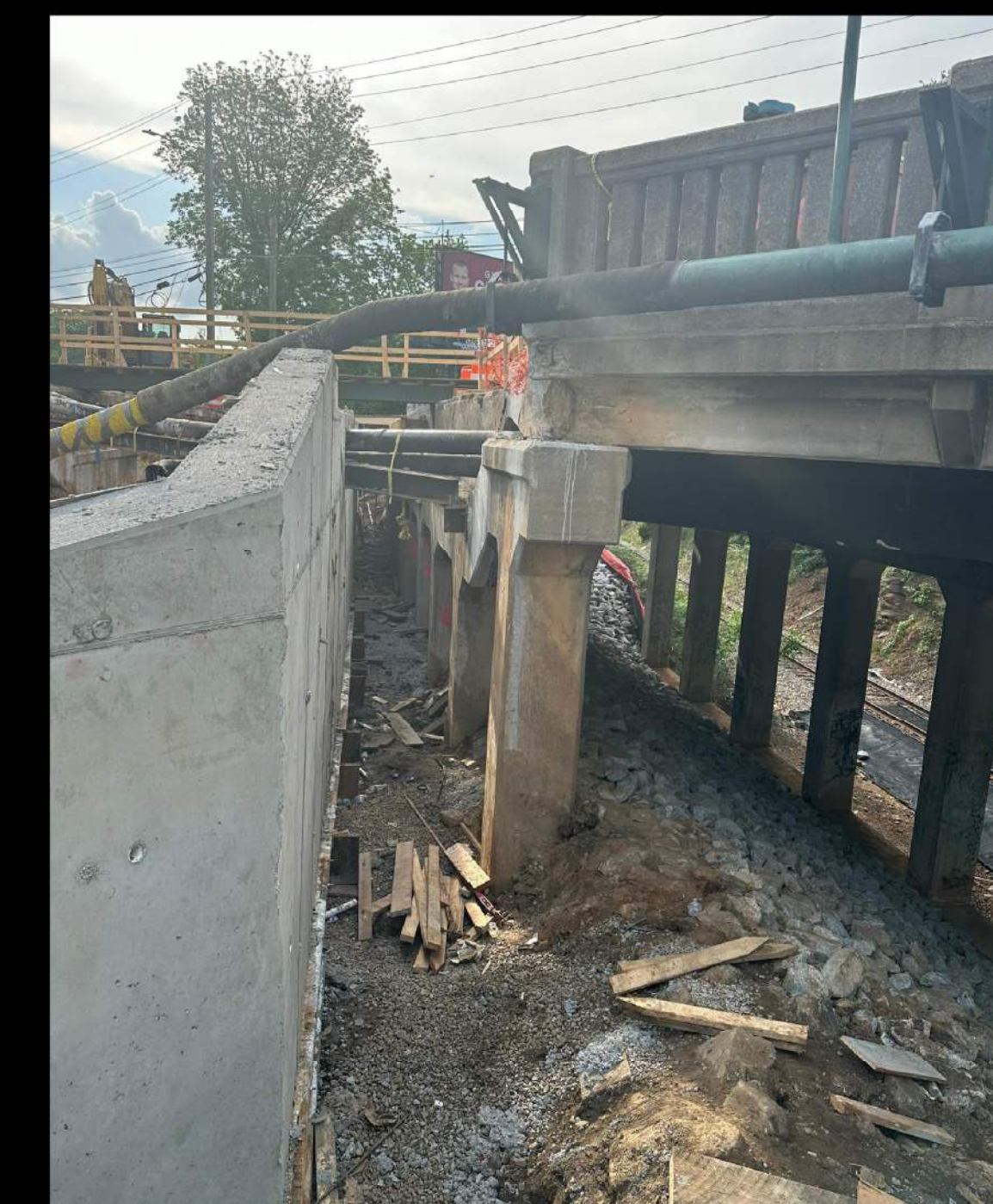
▲ A photo of the vertical abutment wall constructed behind pier with temporary utility supports for gas main and fiber cable ducts.
