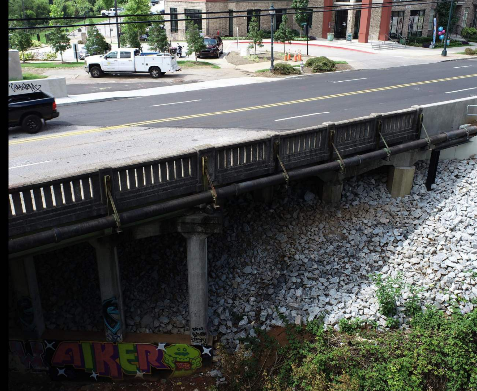
▲ An aerial image of the completed repair showing vertical abutment wall, utility support for 12-inch diameter watermain and column encasement.
