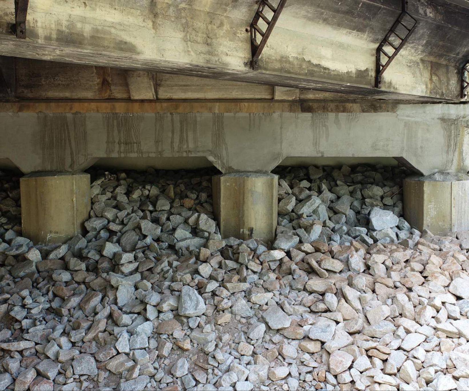
▲ A photo of the cap repair, column encasement and rip-rap placement.
