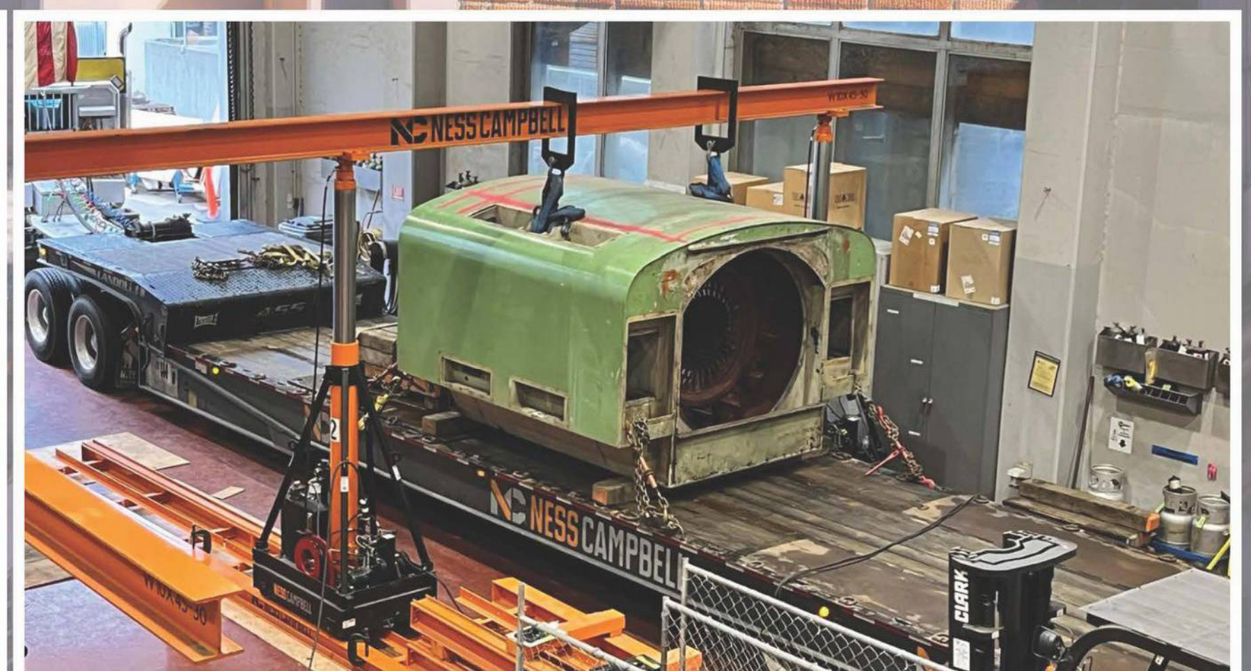
Demolition of the existing steam turbine generator.
