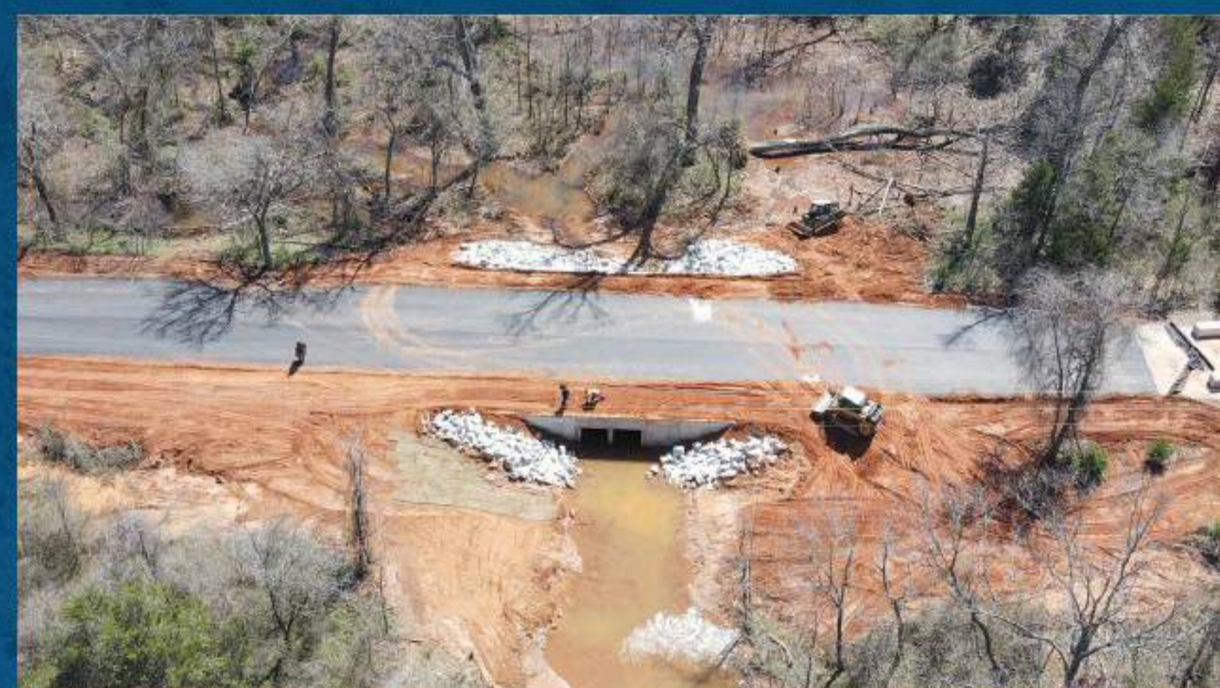
Overhead view showing culvert and roadway installation during construction.
